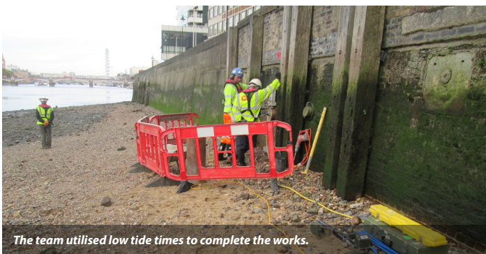
Horizontal coring taking place from the foreshore using a support frame
